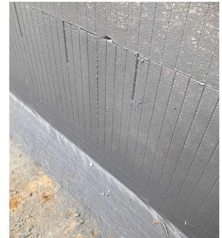
part of a perimeter retaining wall treated with Termseal's Multi-Purpose Active
